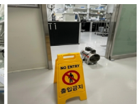
4 Restrict Access to the Site/Provide Forced Ventilation
